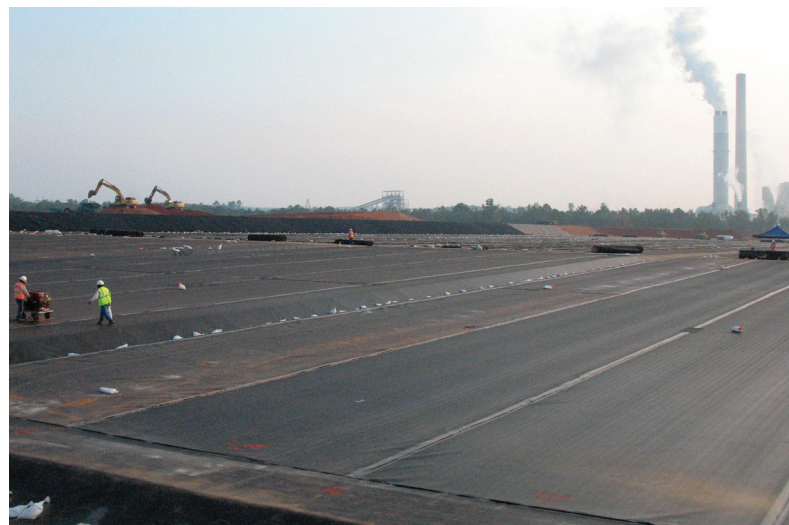
New CCR landfill liner system installation at a Georgia Power plant
