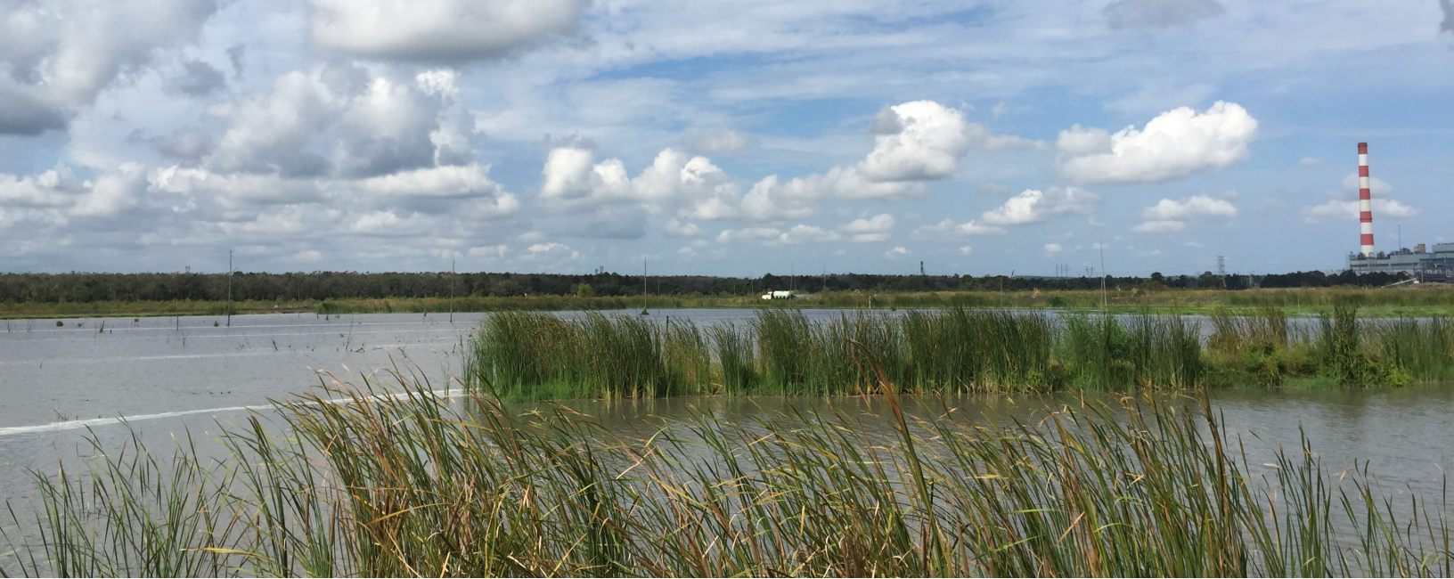
An ash pond in Alabama
