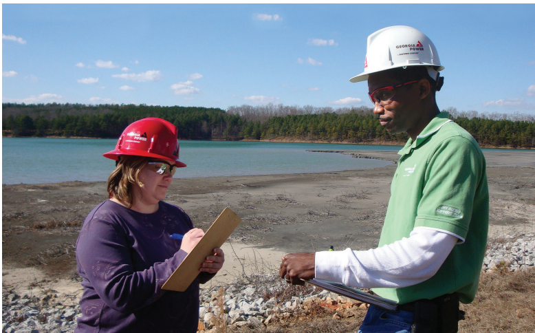
Southern Company system employees inspect a dam, part of the regimen to ensure safety.
